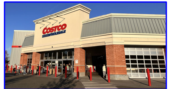
COSTCO - Over 23 Costco Stores Built & Remodeled By Hedley
